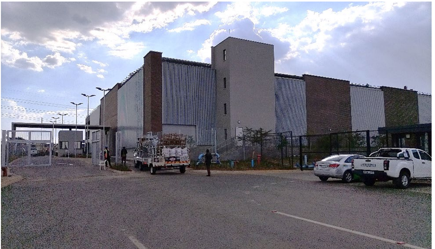
Phase 1 Central Hub 2023/2024
