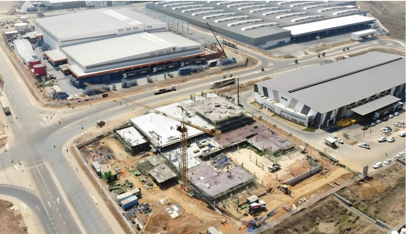
Phase 1 Facilities including Central Hub 07 September 2023
