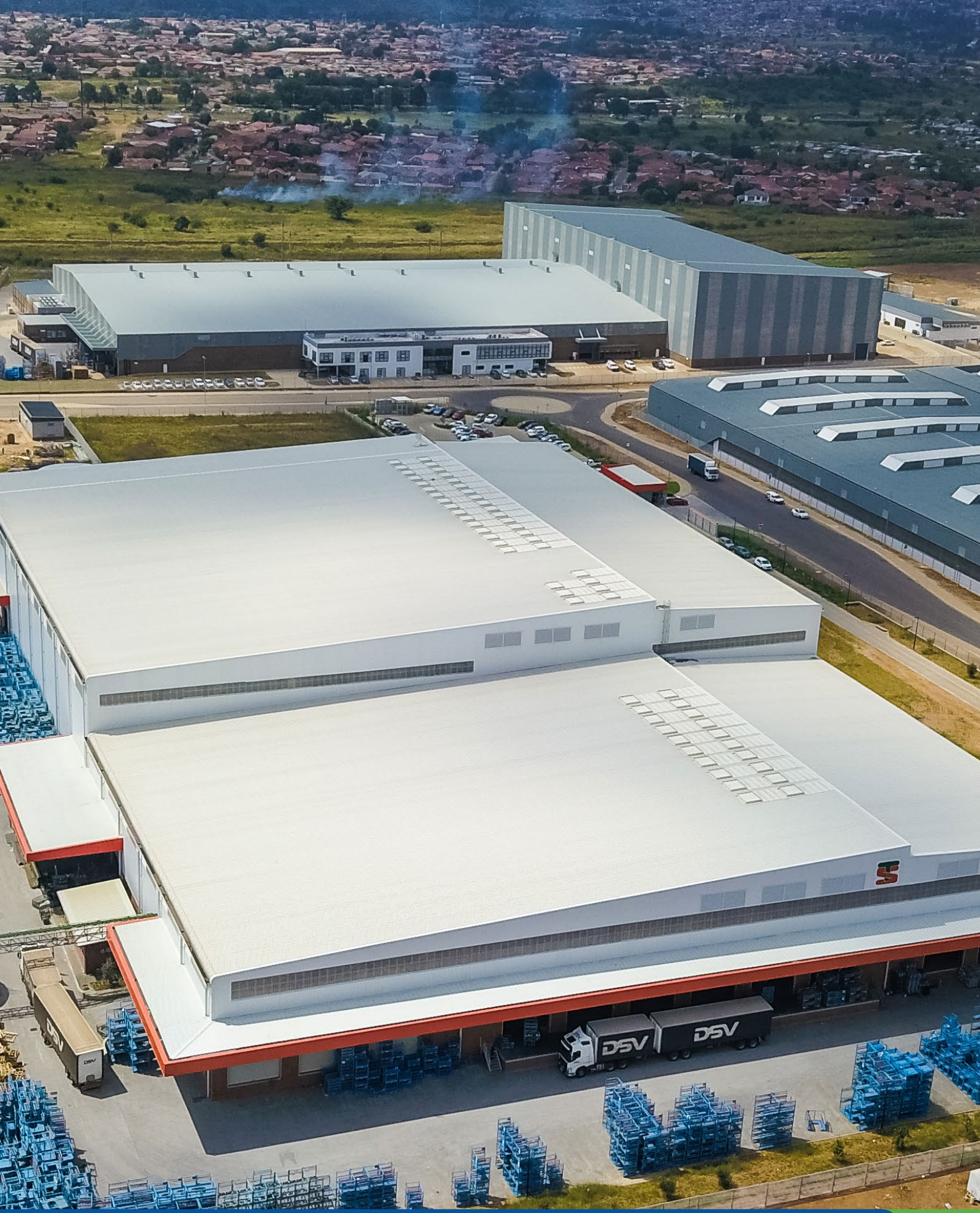
Phase 1 Facilities (Balance of facilities in Phase 1)
